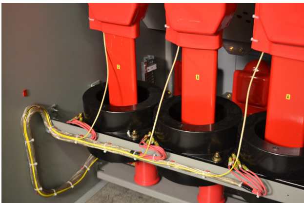
Figure 19: Completed Fiber Installation
