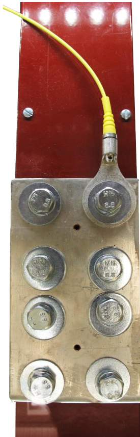
Figure 15: Correctly Installed Probe and Lug
